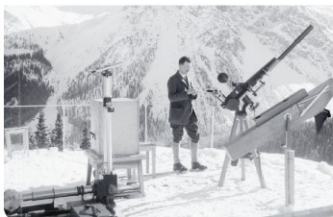
Figure 6: Daniel Chalonge, colleague of F.W. Paul Götz, on the terrace of the 'Finelicht' house in Arosa in the early 1930s, between the Fabry-Buisson (predecessor of the Dobson spectrophotometer), the Chalonge, and the Féry spectrographs. Photo: unknown. Source: Photo archive MeteoSwiss
